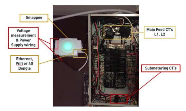
Example of a complete Smappee Plus Installation on a US Split phase (240V) installation with solar and a wiring harness used for voltage measurement and power supply. Ethernet used for internet connection.
