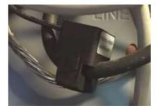
Use one CT on each phase of the load and ensure it has a rating equal to or greater than the breaker rating protecting the circuit (i.e. 200A CT for a main circuit with a 200A breaker rating). Then plug the other end of the CT into the corresponding inputs (1-9) on the Smappee Plus monitor.
