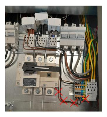
The picture below shows the situation after removing the pre-wired cables:
