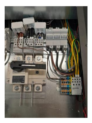
Mount the 5G2.5 mm<sup>2</sup> cable to the connecting block, respecting the colour assignment. The 5G 2.5mm<sup>2</sup> cable is secured with a 2OA circuit breaker in the distribution panel.
