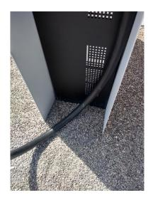
The EV Base Ultra can be placed maximum 3 cm below the top of the surrounding soil for aesthetic purposes. It cannot be placed lower as there will be risk of water ingress.
