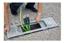
e. Place the EV Base Ultra (with floor plate) over the anchor. Make sure all holes align with sides of the anchor and the power supply and ethernet cables go through the central opening of the EV Base Ultra.
