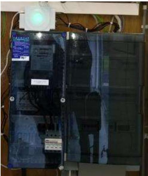
Monitor positioned on top of electric panel
