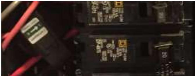
Example of submetering on a Single-Phase 120V circuit
