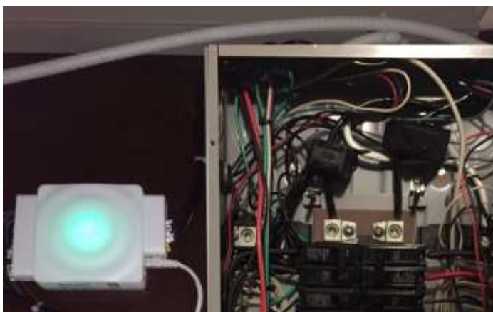
Monitor mounted on wall electric panel
