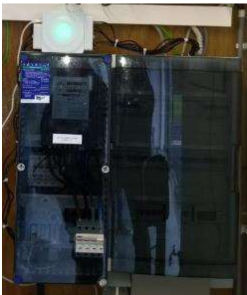
Monitor positioned on top of electric panel
