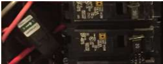
Example of submetering on a Single-Phase 120V circuit
