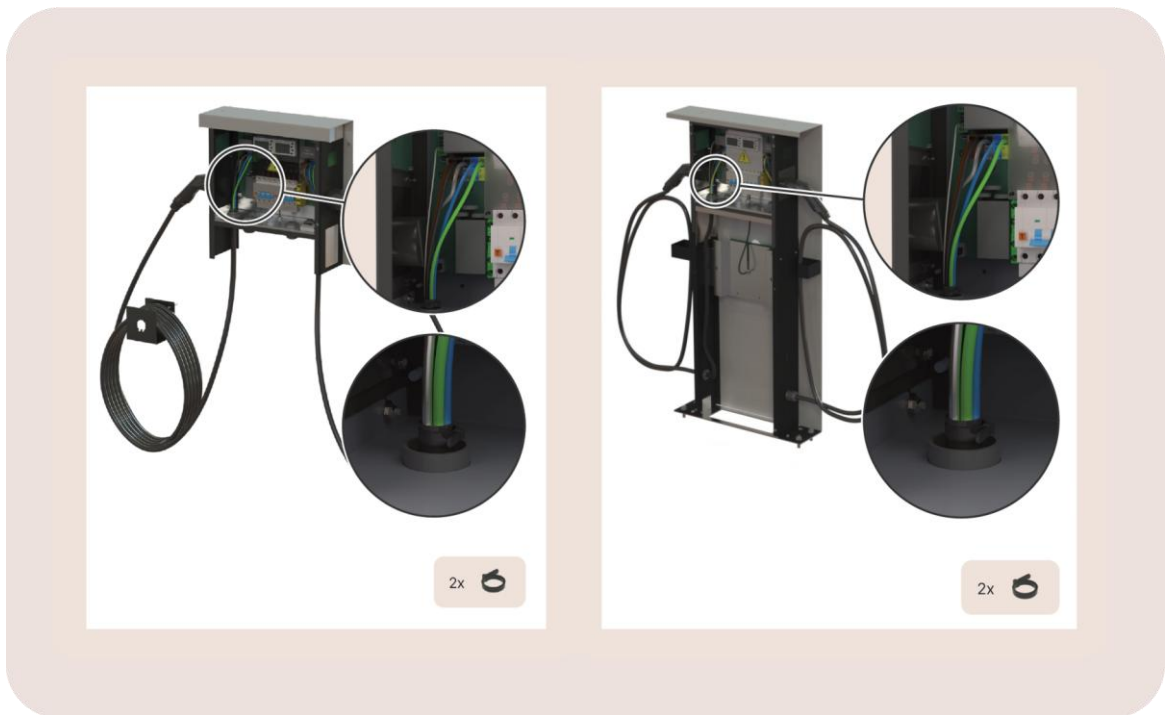
Image 32: View on the cable connections for a wall mounted and ground mounted EV Dual
